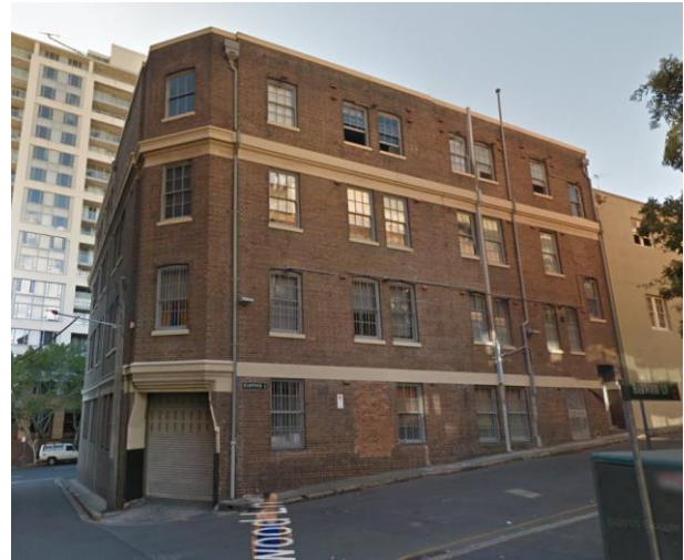
PICTURE 4 – 47 MURRAY STREET LOOKING EAST
