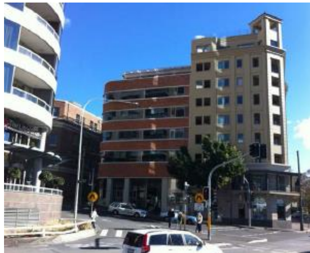
PICTURE 2 – 43 MURRAY STREET LOOKING WEST
